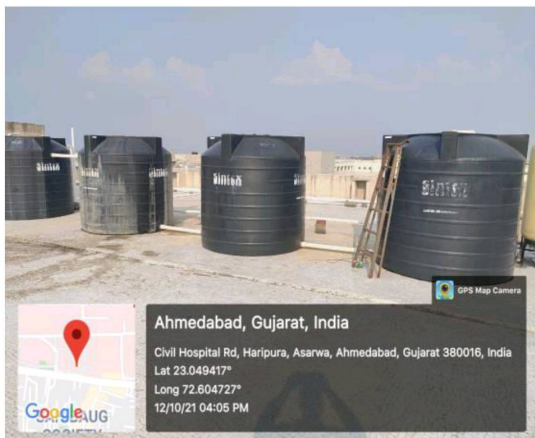
Overhead water tank
